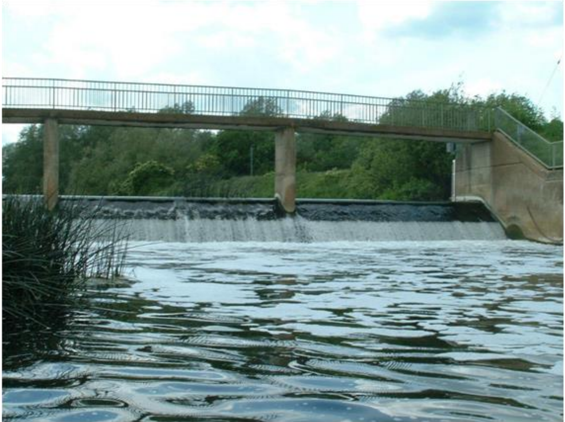
Figure 7.4. Sharnbrook weir, photo taken in an upstream direction.
