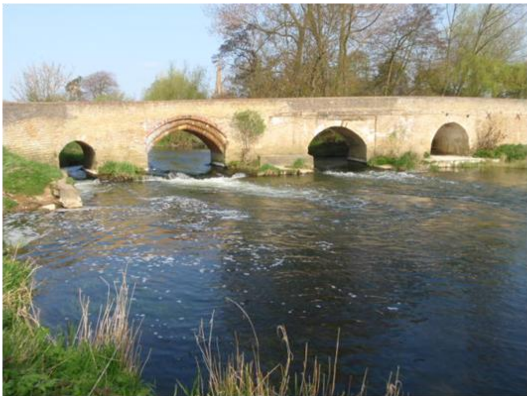
Figure 7.3. Harrold Bridge weirs, photo taken in an upstream direction.
